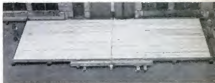
Above, a partially completed model floor frame with spaced diagonal braces laid one way under lengthwise flooring. This construction proved by far the stiffest on exceptionally long floor frames. Below, the finish flooring is laid the long way
